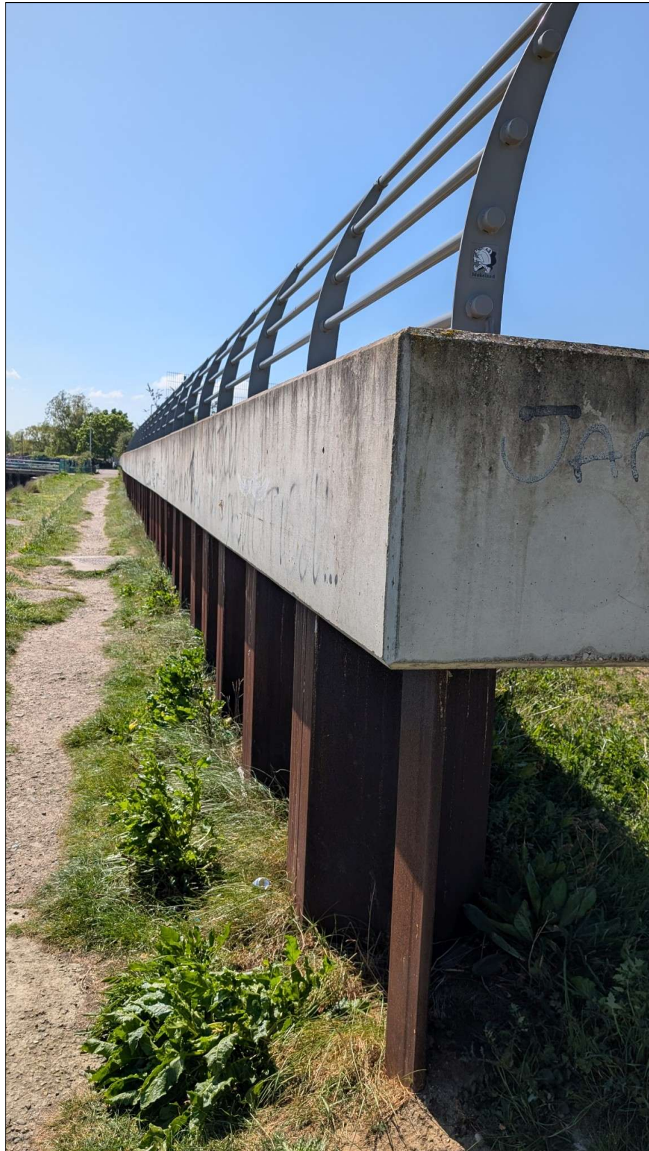
Figure 2-4 Flood defence wall at SNF41.
