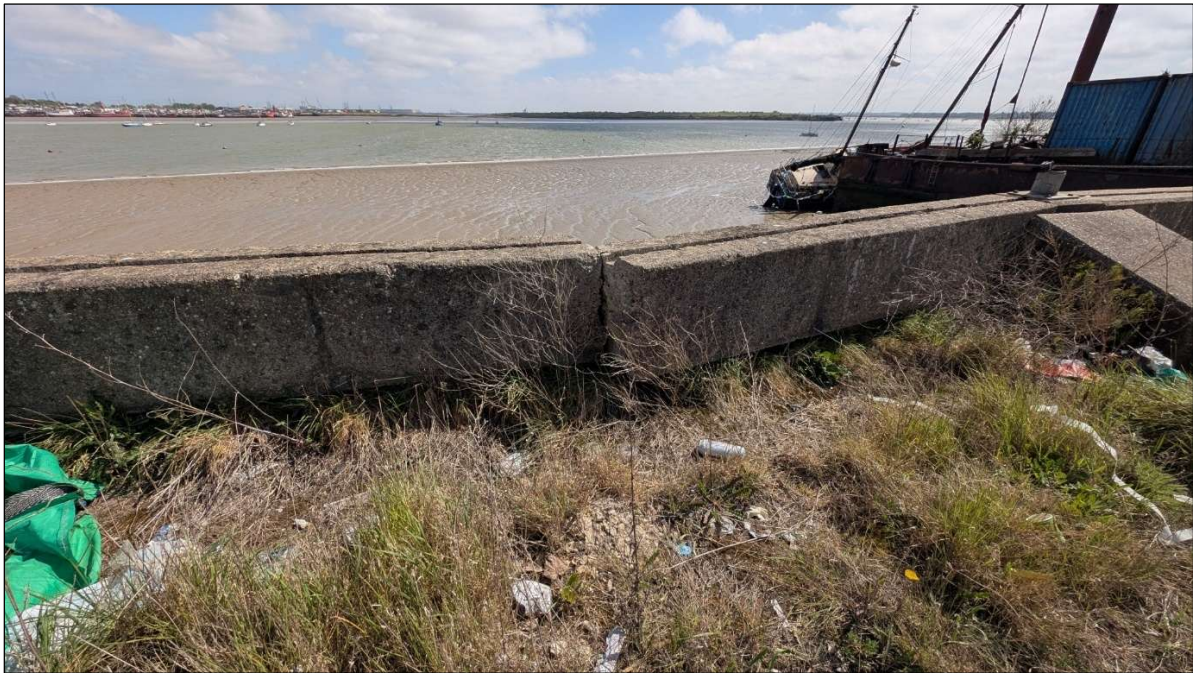
Figure 2-1 Site walkover photographs of the flood defences at SMI6.
